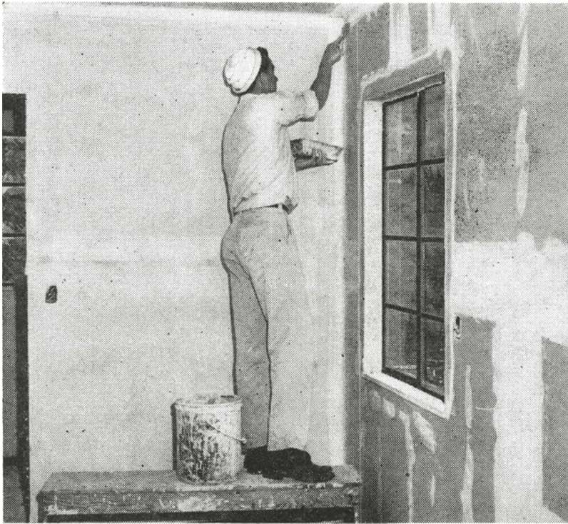
9. A factory craftsman tapes the wallboard seams for smoothness.
