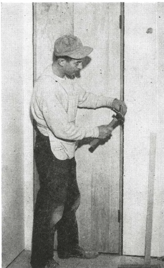
10. Putting in the pre-hung doors is another of the many finishing jobs calling for no professional skill.
