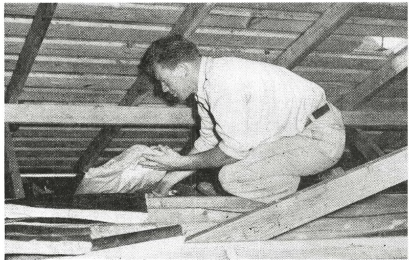
12. A friend of the owner does his bit by installing rock-wool batts between the ceiling rafters for insulation.
